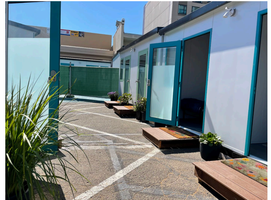
Non-congregate cabin program at 33 Gough.
